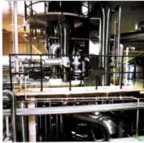
Figure 7 (top left): This Compression heat pump saves energy in timber drying by recycling the expelled heat.
